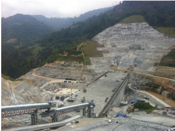
Susu Dam – RCC Construction
