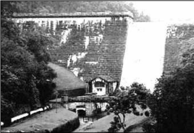
View of Pulau II Dam, Johor
