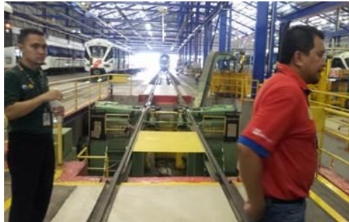
Train maintenance platform
