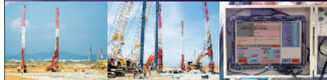
New Low Cost Carrier Terminal (LCCT), Sepang, Selangor.
