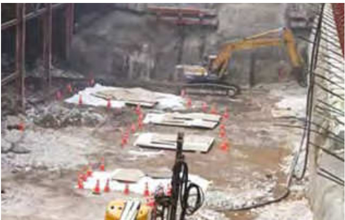
Photo 5: Blast area preparation at Maluri site (after Goh et al., 2015)
