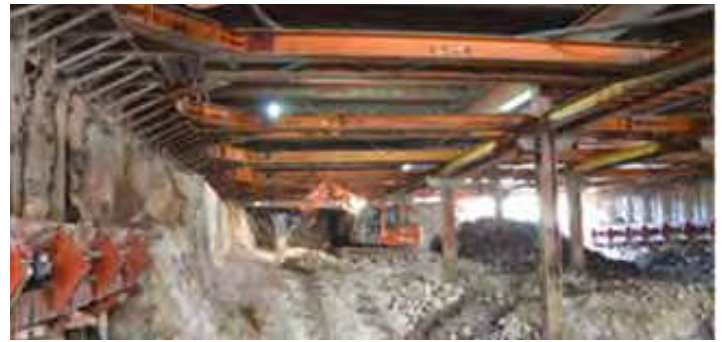
Photo 7: Temporary struts and ground anchors installed in phased sequence of excavation (after Goh et al., 2015)
