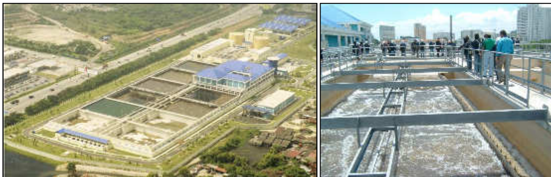
Figure 3.3 : Jelutong Sewage Treatment Plant (1,200,000 PE)
