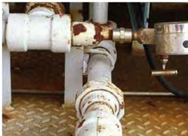
Photo 10: Corrosion In Piping And Fittings
