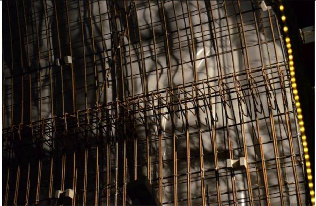
Photo 12 : Reinforcements and water proofing membrane for concrete lining construction
