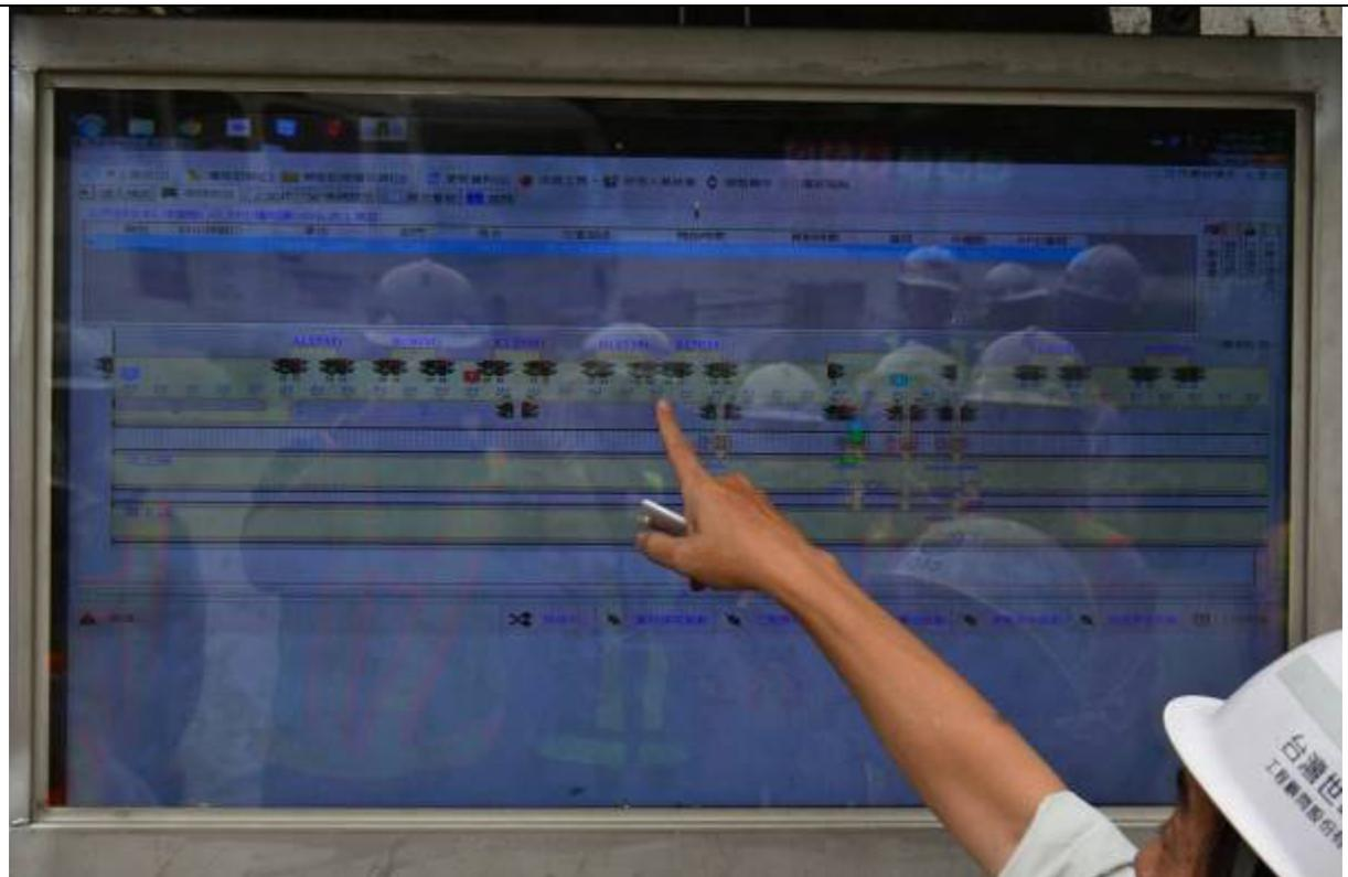
Photo 17 : LCD display at tunnel portal showing locations of workmen and construction vehicles inside the tunnel using RFID
