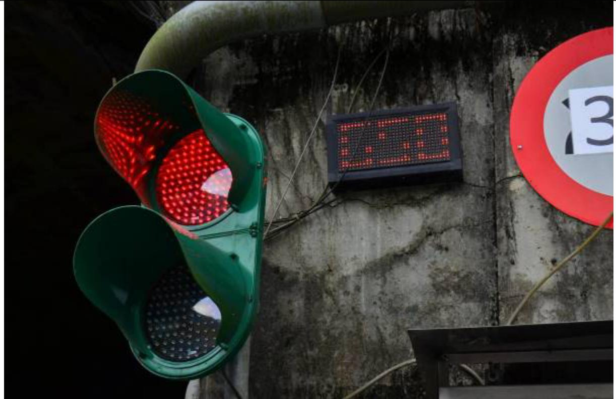
Photo 16 : Traffic signalling with time control using Radio Frequency Identification (RFID) technology for positioning workmen and vehicles inside the tunnel
