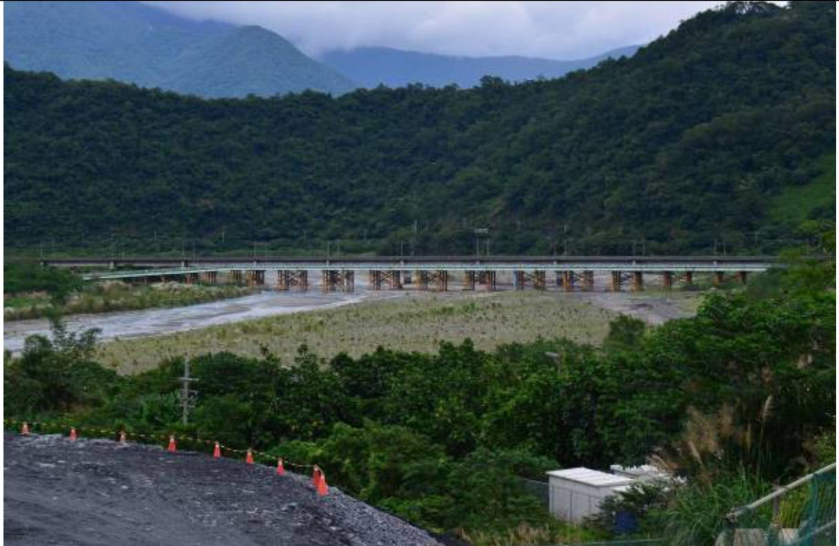
Photo 14 : Temporary steel bridge crossing over stream with primary objective of implementing environmental protection measures
