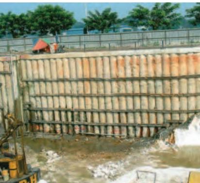
SGE Jacked Anchors for 10-12m CBP Retaining Wall, SMART Tunnel.
