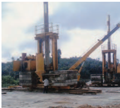
East Coast Expressway, Kerteh, Terengganu Close to 100000m of Stone Column was constructed
