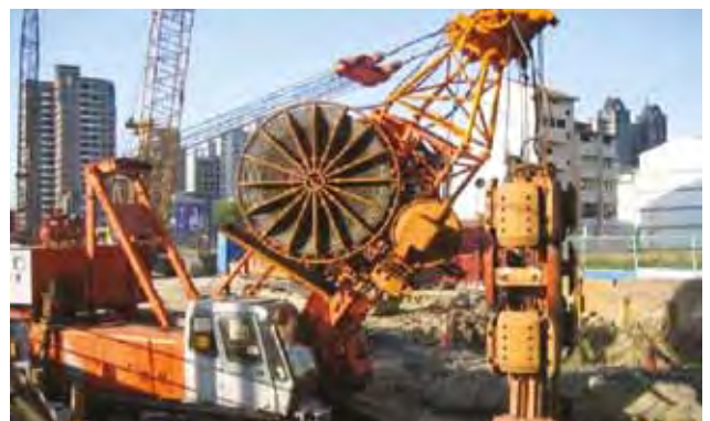
Figure 2: Slurry wall construction with horizontal and vertical site constraints, and modified slurry wall equipment
