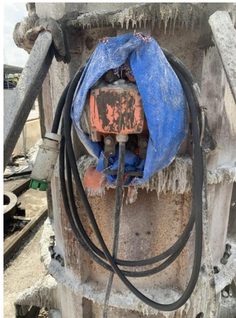
Figure 9: Close-up details of mounting vibrator.
