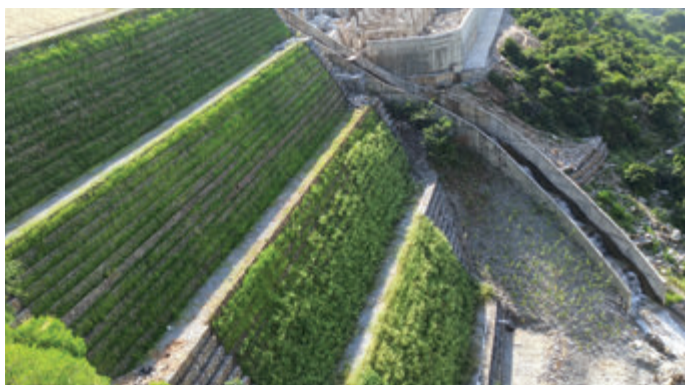
Terramesh® System with Paraproduct geogrids
