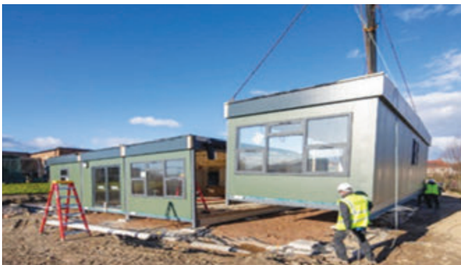
Figure 3: Modular construction as temporary accommodation (elitesystemsrgb.co.uk)
