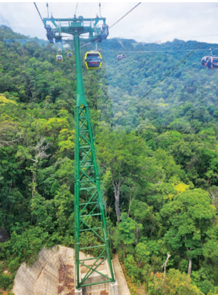
Cable car pylons structures
