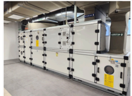
VRV AHU – WITH FULL COMPONENTS: HEATWHEEL, EC PLUG FAN, CONTROL ETC
