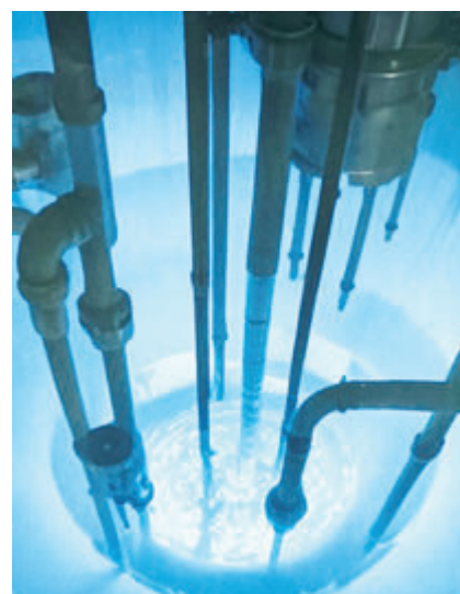
TRIGA PUSPATI Reactor core submerged in distilled water that serves as a neutron coolant and moderator
