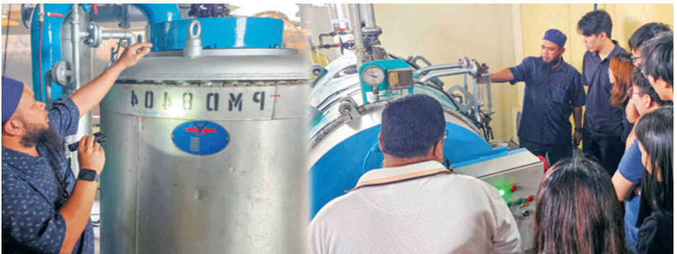
Mr. Hiswandy explaining how chemical treatment is applied to once-through steam boiler
