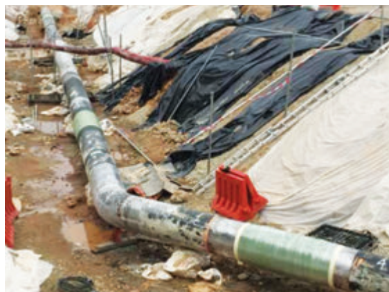
General overview of pipeline with composite wrapping system (iWrap® 100N)
