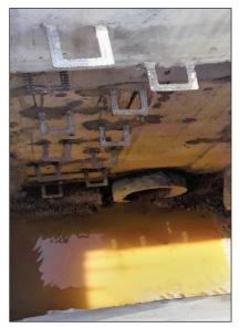
Figure 5.2 Water ponding issue in manhole or inspection chamber due to mismatch invert level
