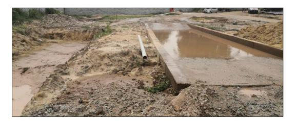
Figure 7.3 Untreated Backfilling and Washing Bay
