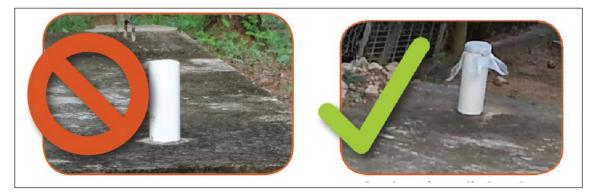
Figure 5.11 Exposed vent pipe shall be properly seal with screen mesh (Source: Department of Health and Human Services-US)
