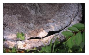
Figure 5.3 Broken septic tank cover
