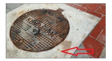
Figure 5.9 Manhole or inspection chamber overflow with surface runoff (during construction)
