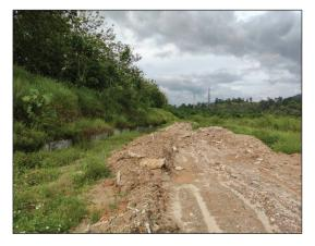
**Uneven Backfilling with Water Ponding**
