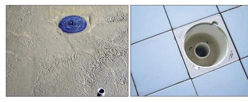
(a) Floor trap cylindrical body cast to the floor slab with a cover.
