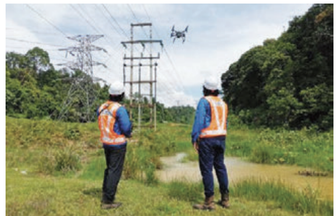
Figure 1: The application of UAS in the regime maintenance of overhead lines in TNB Distribution Network
