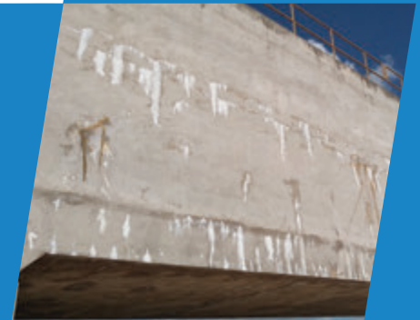
Xypex crack self-healing capability can be seen on the exterior of the aqueduct.
