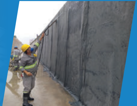
Curing of Xypex Concentrate in hot conditions.
