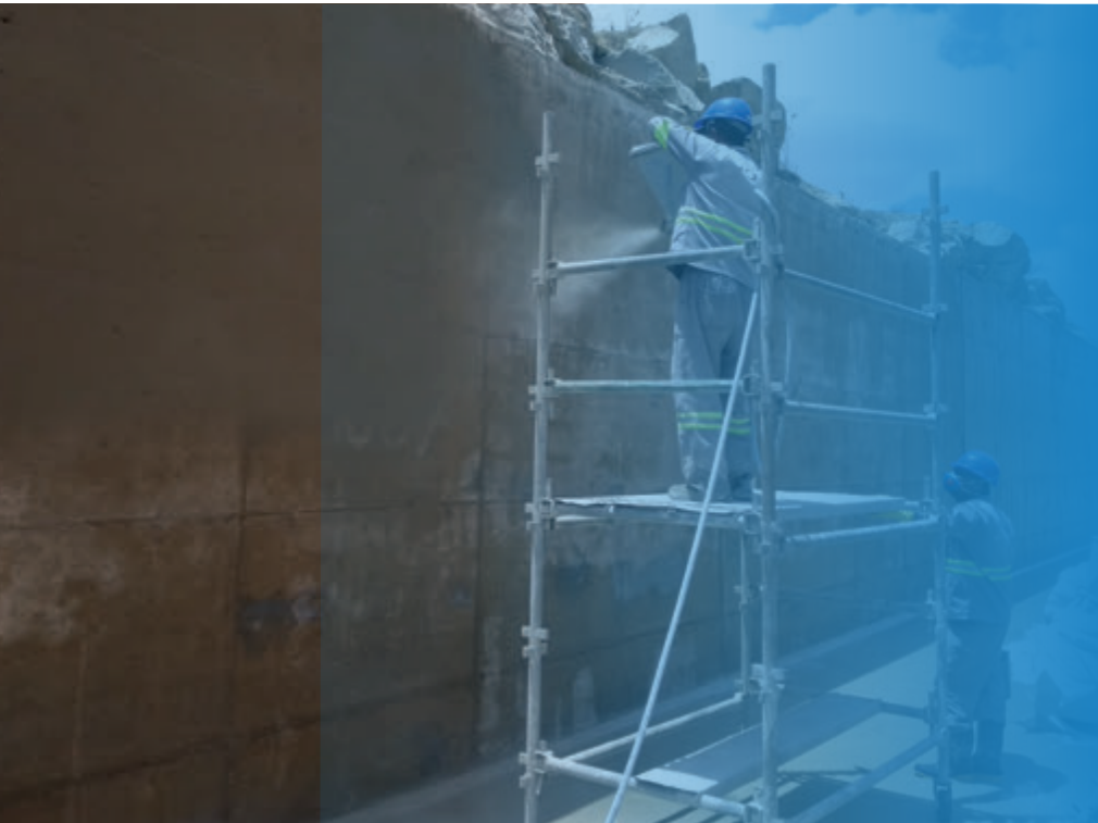
Application of Xypex Concentrate using a hopper gun.
