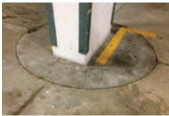
Figure 2: Round isolation joint
