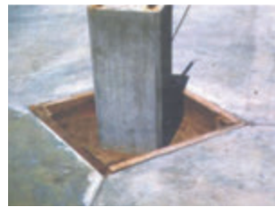
Figure 3: Square isolation joint
