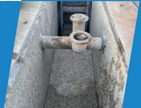
Severe damage in the concrete caused by Microbial-Induced Corrosion (MIC).
