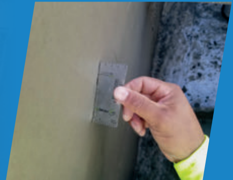
To ensure the performance, the resurface's thickness was verified throughout the process.
