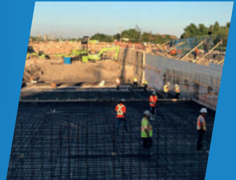
Xypex was added to the concrete to create a waterproof barrier
