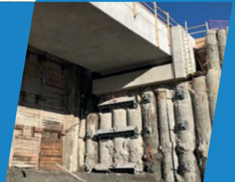
The secant piles were treated with Xypex Admix
