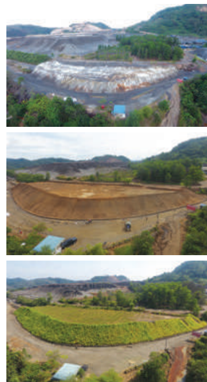
Figure 1: Pictures showing 3 stages of how the "encapsulation technique" is used to treat the acid mine drainage issue.
