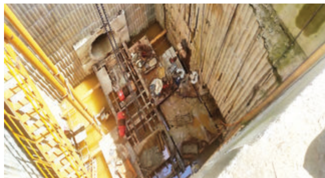
Figure 2.2: Hard ground was cored and used as a shaft wall in Langat, Kajang
