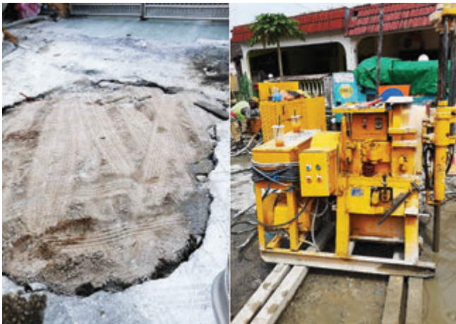
Figure 2.3 (d): Rectification of the settlement road with backfilling, concrete and pressure grouting at manholes along Jalan Kapit, Taman Beringin
