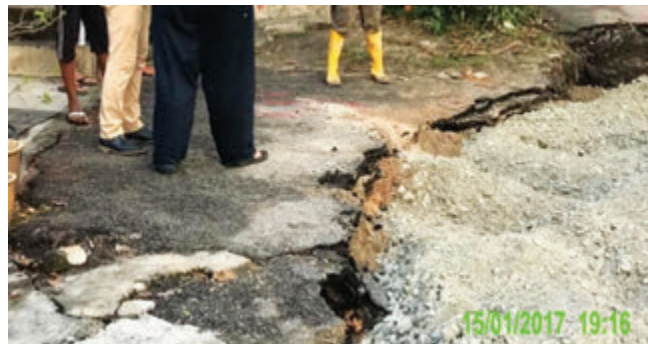
Figure 2.3 (a): Road settlement at manhole N-19, Jalan Bintulu, Taman Beringin
