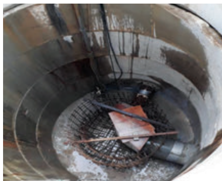
Figure 1.1: Concrete Caisson Shaft construction at Hulu Langat, Kajang
