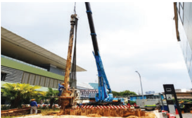
Figure 2.4(a): Shaft next to the office building installed by using silent piler at Pakej D49, Kajang
