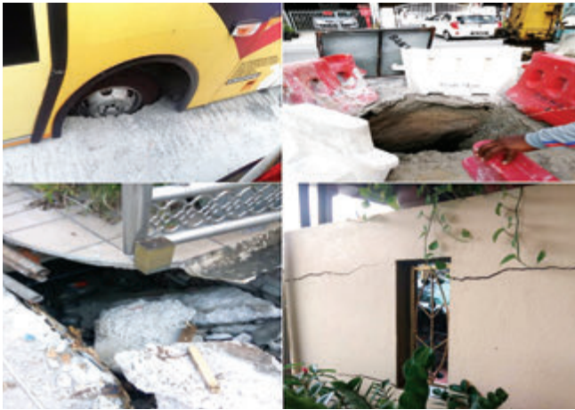
Figure 2.3 (c): Sinkhole at manhole N-17 (Zone 3B) along Jalan Kapit, Taman Beringin
