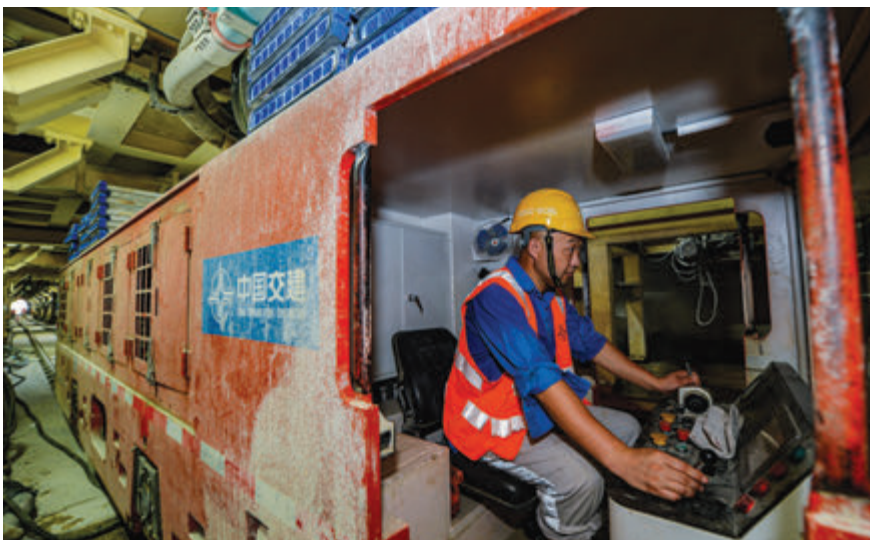
A locomotive operator transporting materials to the Tunnel Boring Machine, Genting TBM1
