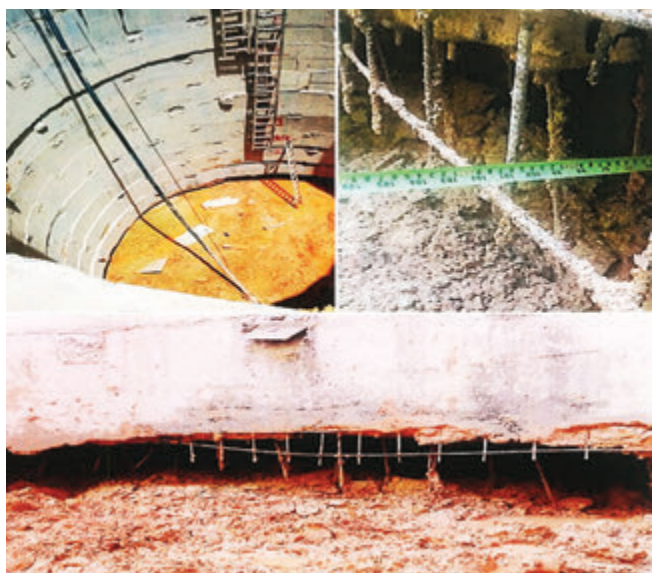
Figure 2.0: Shaft bottom soil collapsed. Concrete grouting was applied to stabilise the soil at Hulu Langat, Kajang
