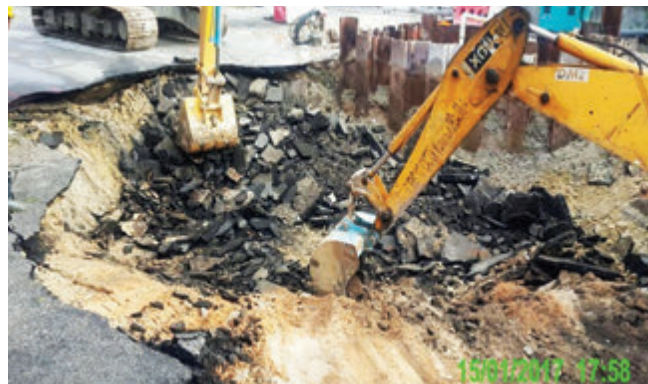
Figure 2.3 (b): Road settlement at manhole N-19, Jalan Bintulu, Taman Beringin
