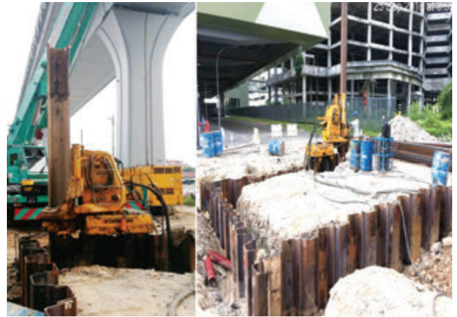
Figure 2.4(b): Shaft next to highway pier installed by using silent piler at Pakej D49, Kajang
