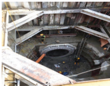
Figure 1.0(a): Sheet pile Cofferdam Shaft construction at Langat Cheras, Kajang
