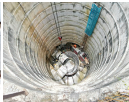
Figure 1.2: Cast-in-situ concrete shaft construction at Hulu Langat, Kajang
