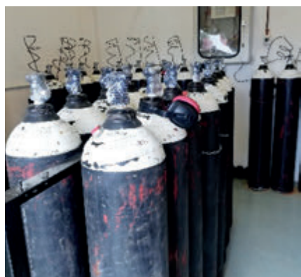
Figure 2: Oxygen cylinders and manifold
