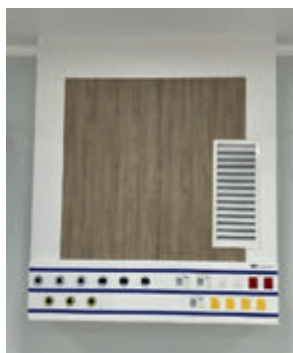
Figure 5: Bed head panela with medical gas terminal units in the field hybrid ICU
