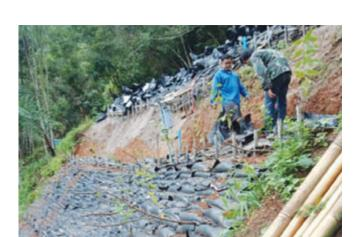
Figure 2: Flapped soil bags with live stakes and micro-piles (Dr Apiniti's slide)
