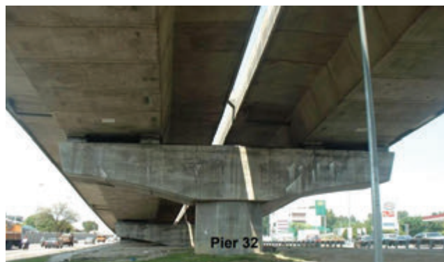
Figure 1: Pier 32, one of the 31 T-shape concrete piers that showed cracks
