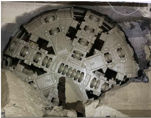
Figure 1: Final TBM Breakthrough at Singapore MRT project.
