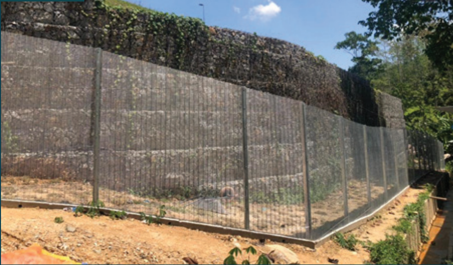
Retaining Wall and Soil Reinforcement
