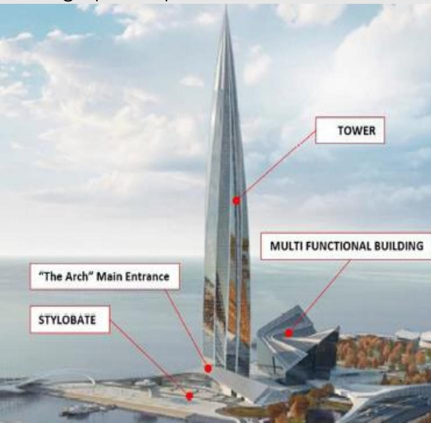
While each of the MFCD buildings is technically challenging in its own right, the focus of this talk is to present the development and integration of the structural and foundation systems of the bowed, tapered, and twisted shape of the tower into the fabric of the tallest Tower in Europe.
