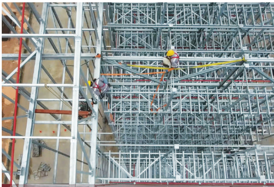
Skywalkers installing warehouse rackings. These specialist workers are trained to work at heights without scaffolding but they are securely fastened with a harness
