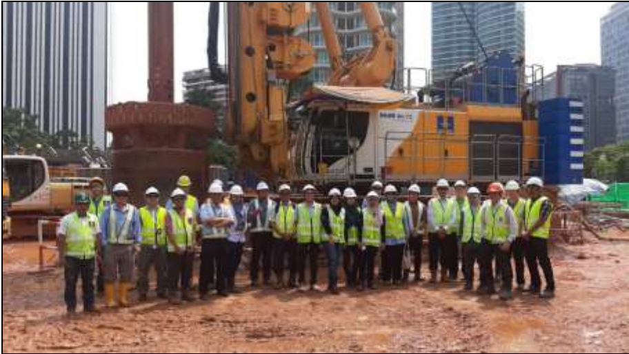
Figure 3: Group Photograph in front of boring rig Bauer BG 72
