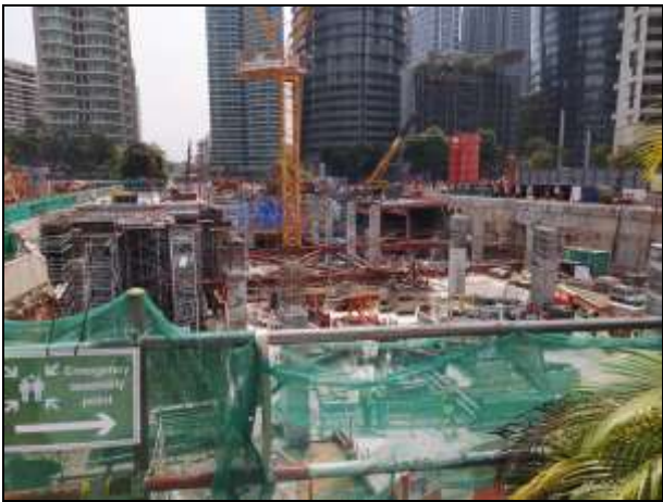
Figure 2: Ongoing Basement Works at 6-Storey Retail Podium Plot
