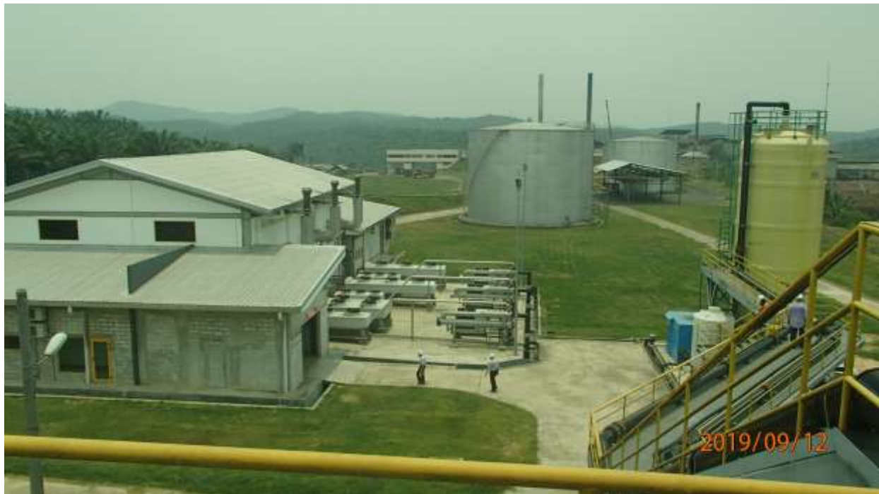
Biogas treatment (de-sulphurization and de-humidification) and treated biogas utilization (power generation for Feed-in-Tariff)-2MW (phase 1) and 1.3 MW (phase 2)
