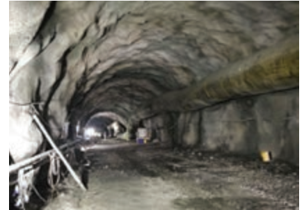
Figure 7: Fibre reinforced shotcrete lined rock face
