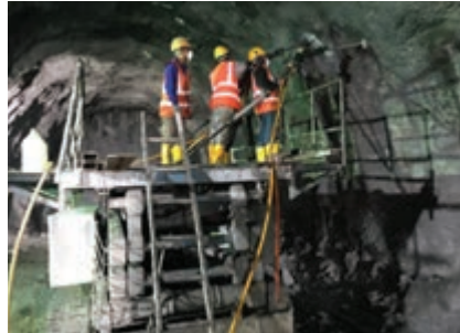
Figure 6: Rock dowel installation
