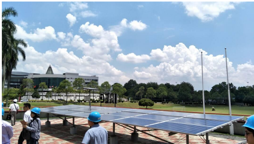
Figure 5: Rooftop of IREC. Wind direction, irradiation level, cell and ambient temperature are being monitored.
