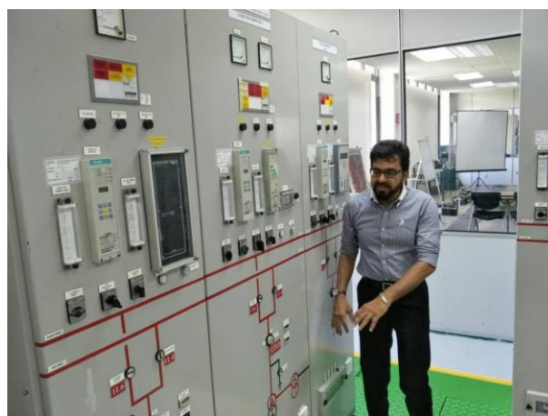
Figure 3: Demonstration of power system protection scheme
