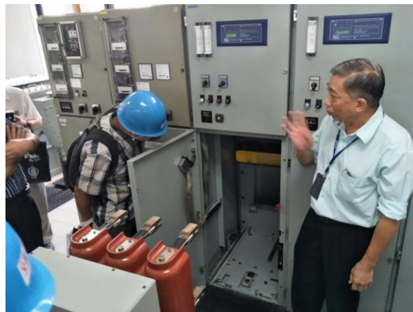
Figure 2: Mr. Mok demonstrating the procedures of safe switching
