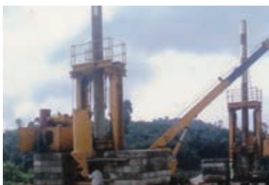
East Coast Expressway, Kerteh, Terengganu Close to 100000 of Stone Column was constructed
