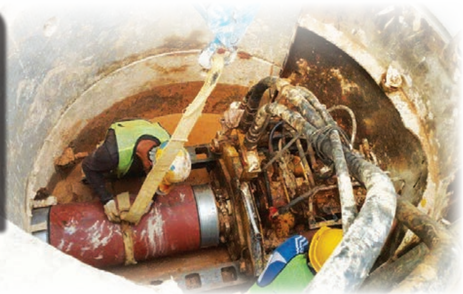
Pipe jacking work in progress
