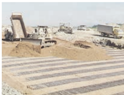
Malaysia's first application of geogrid in Jitra-Butterworth Expressway (1985)
