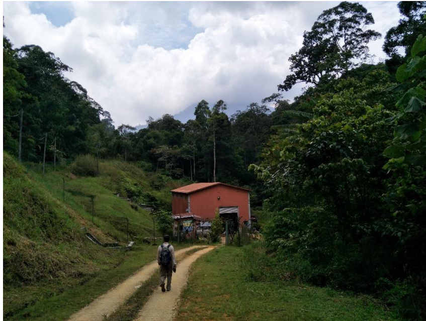
Figure 2: The mini hydropower plant
