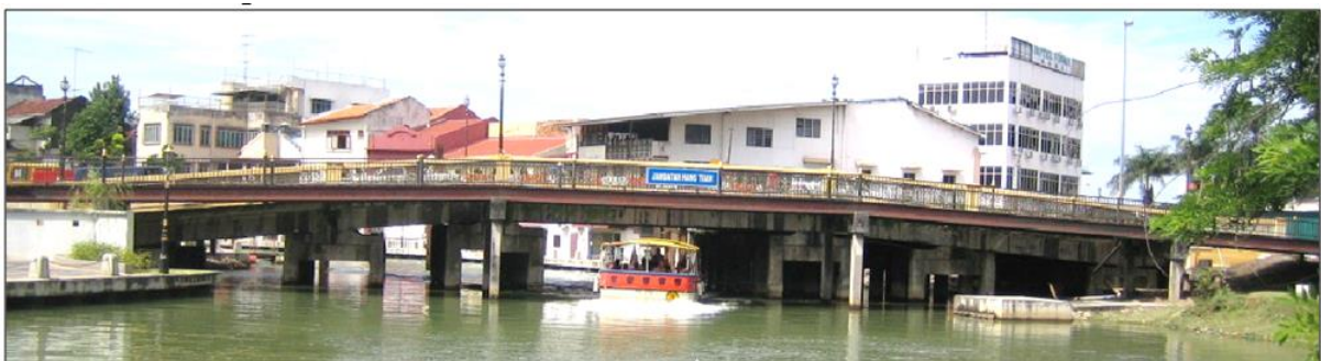
Figure 3: The old 3-span bridge over Melaka River
