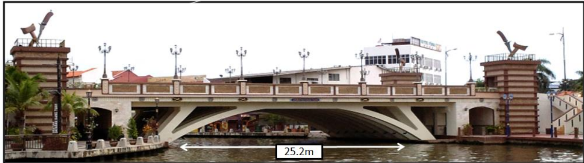
Figure 4: Open spandrel arch bridge over Melaka River
