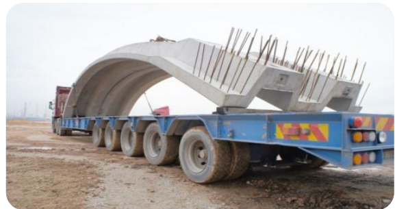
(b) Newly developed and patented corrugated section
