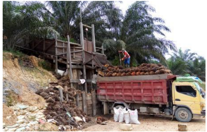
20 tons timber loading ramp (North Kalimantan, 2016)
