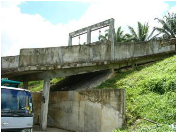
45 tons RC loading ramp (Suai, Sarawak, 2006)
