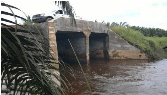
RC box culverts (Sampit, Kalimantan, 2016)
