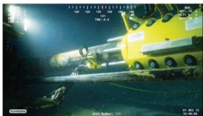
Subsea repair clamp installed by ROV
