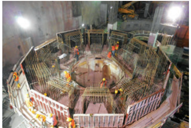
Concrete work around the turbine opening
