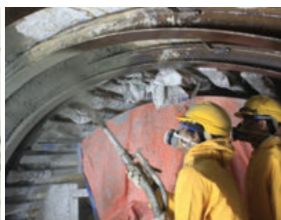
Application of fibre mortar shotcrete behind TBM (Picture courtesy of T. Matsumoto)
