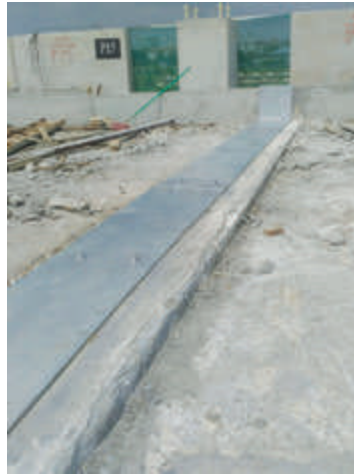
Galvanized Steel Plate Fixed Over to Protect FLEXJOINT EP
