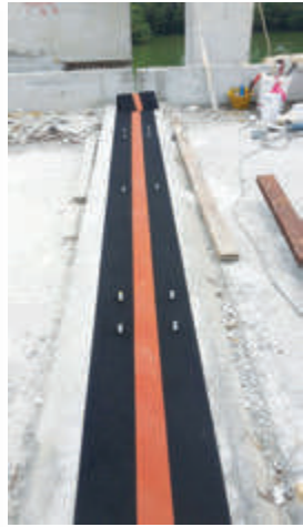
FLEXJOINT EP Laid Over Expansion Joint for Waterproofing
