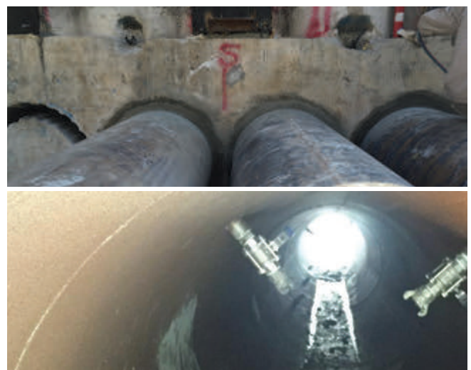
Figure 9: Top: Sealing of the annulus gap between the SBP and the pipe using concrete; One-inch ports inside the pipe used to inject bentonite during excavation and annulus grouting
