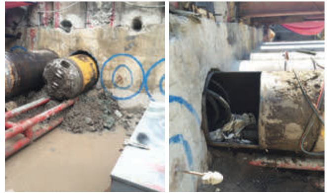
Figure 8: Left: Breakthrough of MTBM at retrieval shaft; Right: Opening for disconnection of umbilical hoses and slurry lines
