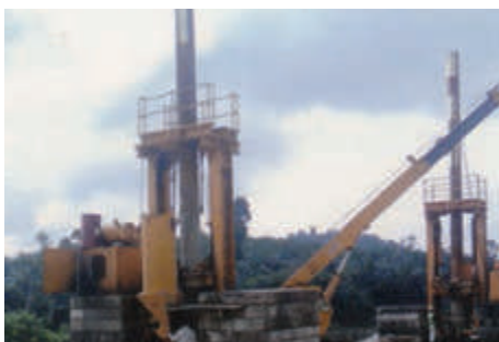
East Coast Expressway, Kerteh, Terengganu Close to 100000m of Stone Column was constructed
