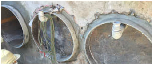
Figure 10: Steel plates were used as end caps for the pipe. Grout was pumped via 2 inch ports welded to the top of the end caps
