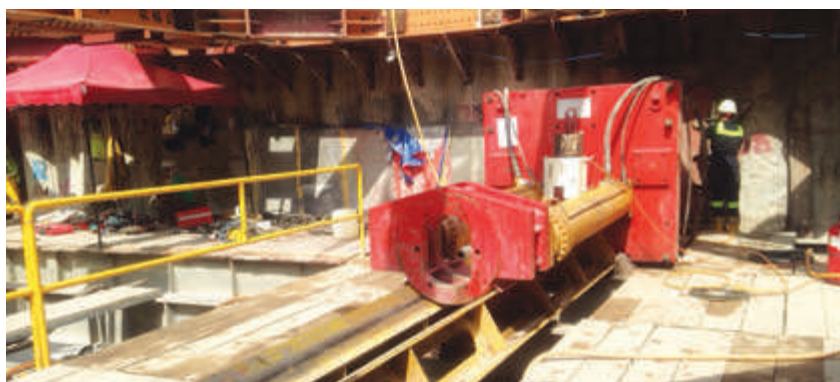
Figure 5: The setup of the jacking frame had to be done for each individual drive
