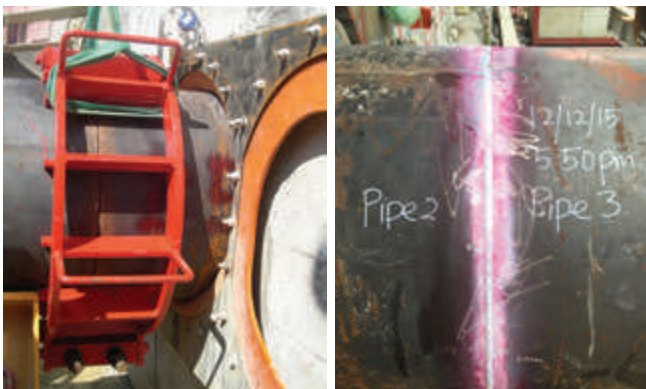
Figure 7: Left: Clamping fixture to ensure concentricity of pipes before welding; Right: DPI testing on completed welds
