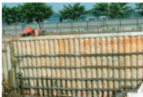
SGE Jacked Anchors for 10-12m CBP Retaining Wall, SMART Tunnel
