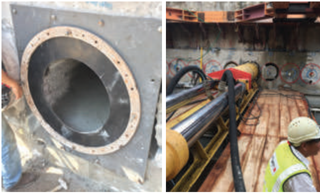
Figure 6: Left: Installed launch shield with rubber gasket; Right: MTBM being launched in the cored SBP
