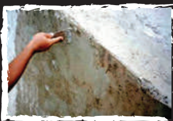
Uneven surface treated with 103 LANKOWALL as patch repair
