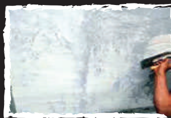
Or apply 103 LANKOWALL as a thin render paste to fill the defects
