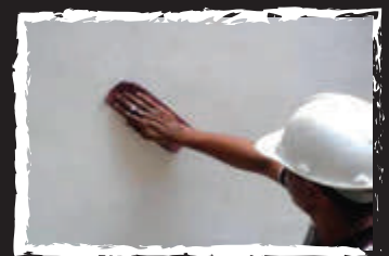
Trace of steel trowel can be smoothened with sandpaper after one day
