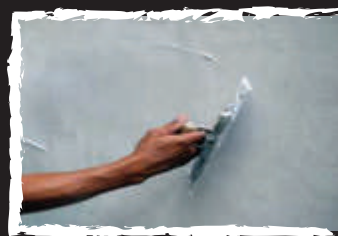
Allow previous layer to dry before applying one more layer as finished surface
