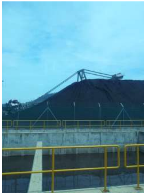
Figure 4: The coal is sourced mainly from Indonesia
