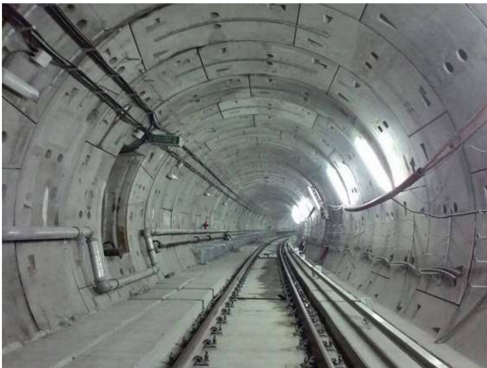
All KVMRT Line 1 SFRC tunnels completed on 11 April 2015
